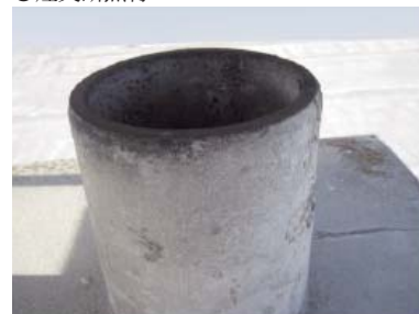
●煙突断熱材
